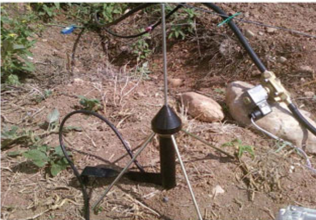
Fig. 2. Valve and UGPA-434 R antenna
